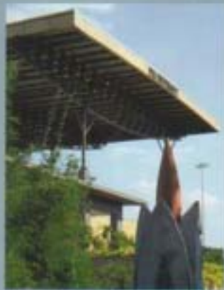
the parasol roof lined with photovoltaic cell to generate electricity
